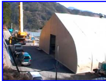
(Placement of crane vehicle)
