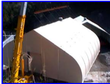
(Moving while hoisting)
