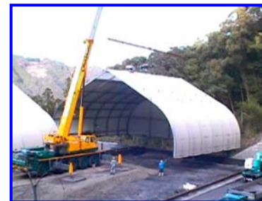
(Moving while hoisting)
