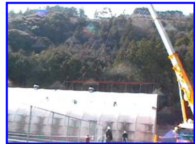
(Attaching hoisting device)
