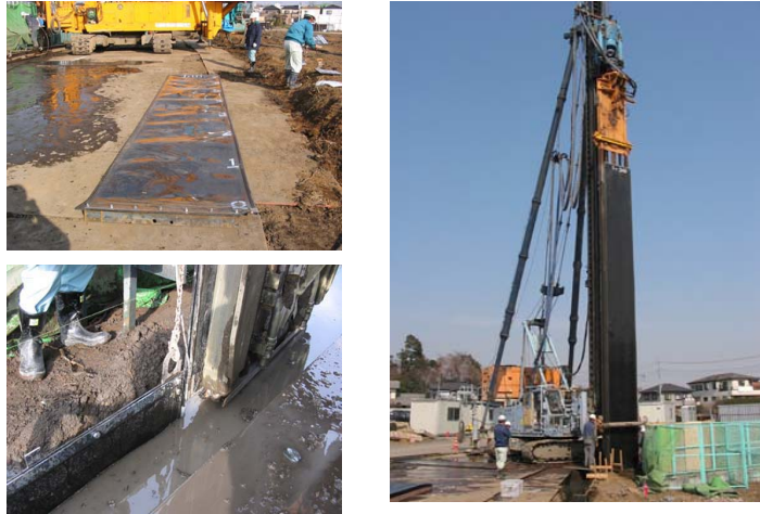
Figure 11. Vertical wall sheeting method
